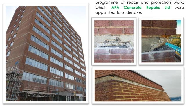
**The solution:** Specified areas of defective concrete were first marked out and subject to saw cutting and breakout, before exposed steel reinforcing was cleaned and protected using Fosroc Nitoprime Zincrich. Fosroc Nitobond HAR was then applied to the prepared concrete substrate, prior to applying Fosroc Renderoc HB to reform the defective concrete, with the finish ensured to match that of the original profile. The ring beams on all elevations were jet washed to readily
